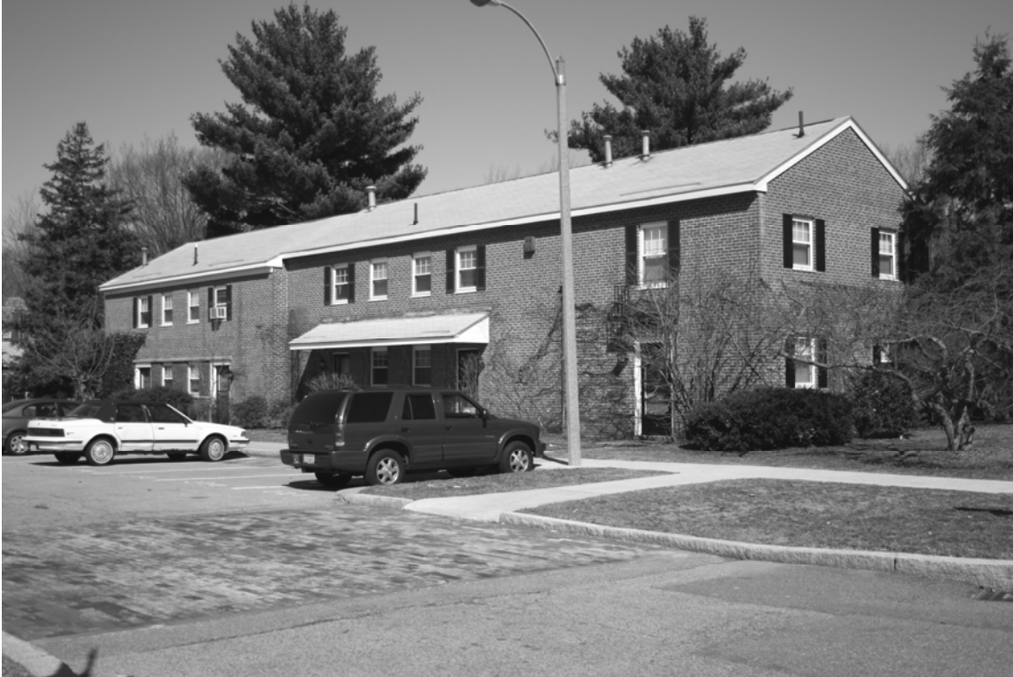
Photo 4 (top, 1 through 9 Gerry Road) and Photo 5 (bottom, 141 through 133 Independence Drive)
