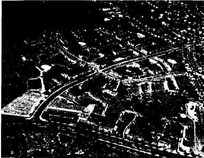
AERIAL VIEW HANCOCK VILLAGE
