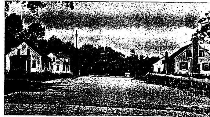
CUSHING ROAD July, 1945
