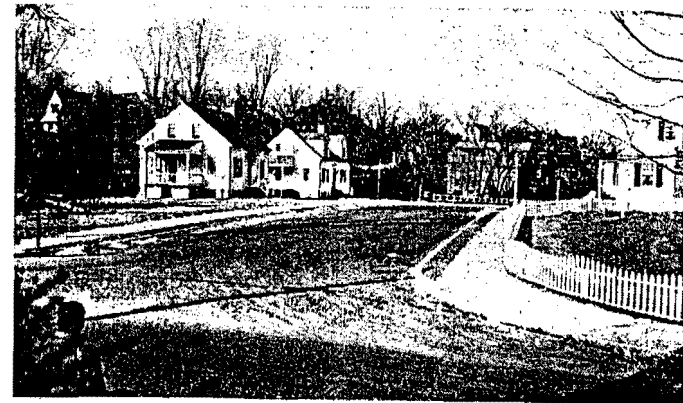
CUSHING ROAD After Construction January, 1946
